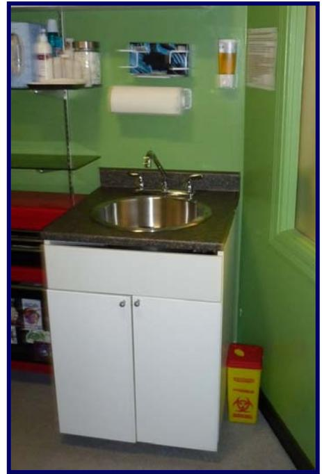
**Figure 1. Stainless Steel Sink for Handwashing and Instrument Reprocessing**
